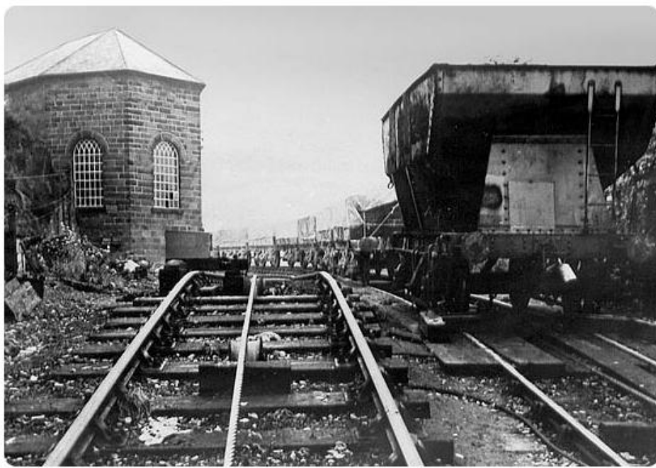
The head of the incline with the winding house in view.
