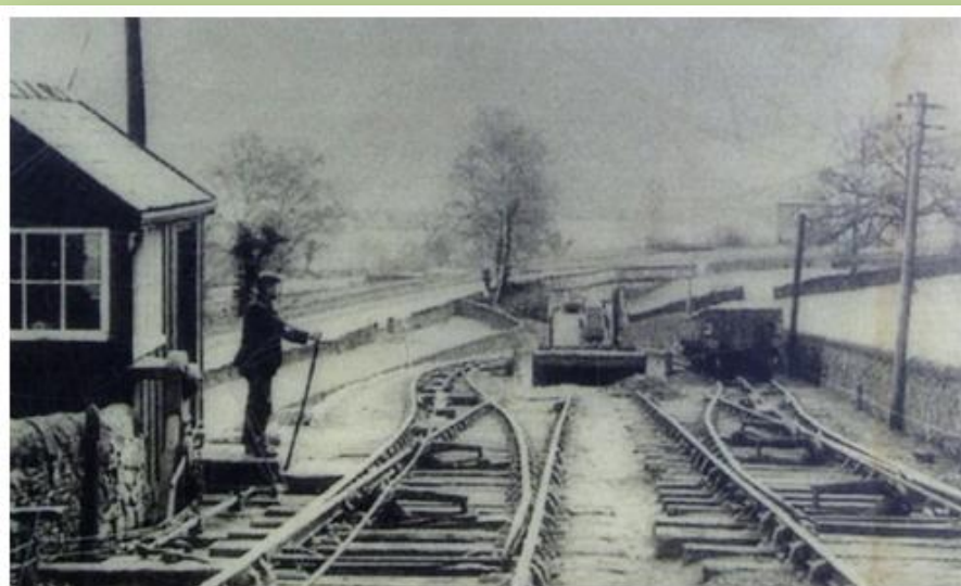
Photograph taken around the turn of the century showing the points which directed runaway wagons into the Catch-Pit.
