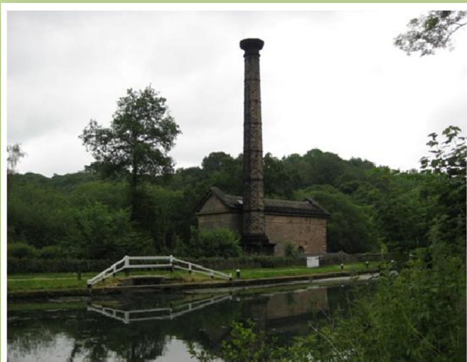
The Leawood Pump House. Note the white fencing. This stands over the point at which water was let into the canal. The water concerned was taken from the River Derwent (directly behind the pump house), and pumped out and into the canal at this point.
