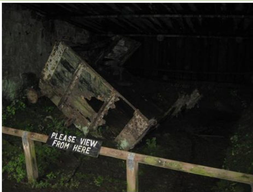
In the Catch Pit, the rusting remains of the last accident on the incline in the 1960's.
