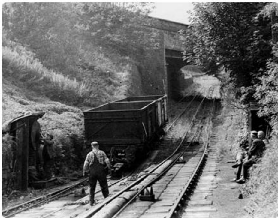
The foot of the incline with the 'Catch Pit' just beyond the tunnel.
